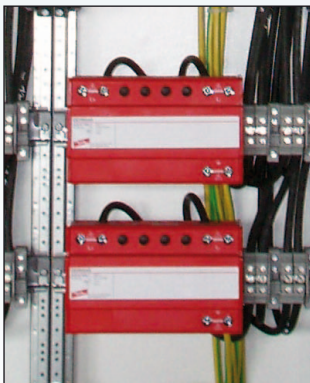
Figure 1.1 Combined arrester Type 1, DEHNlimit PV, to protect photovoltaic inverters from surges also in case of direct lightning strikes
